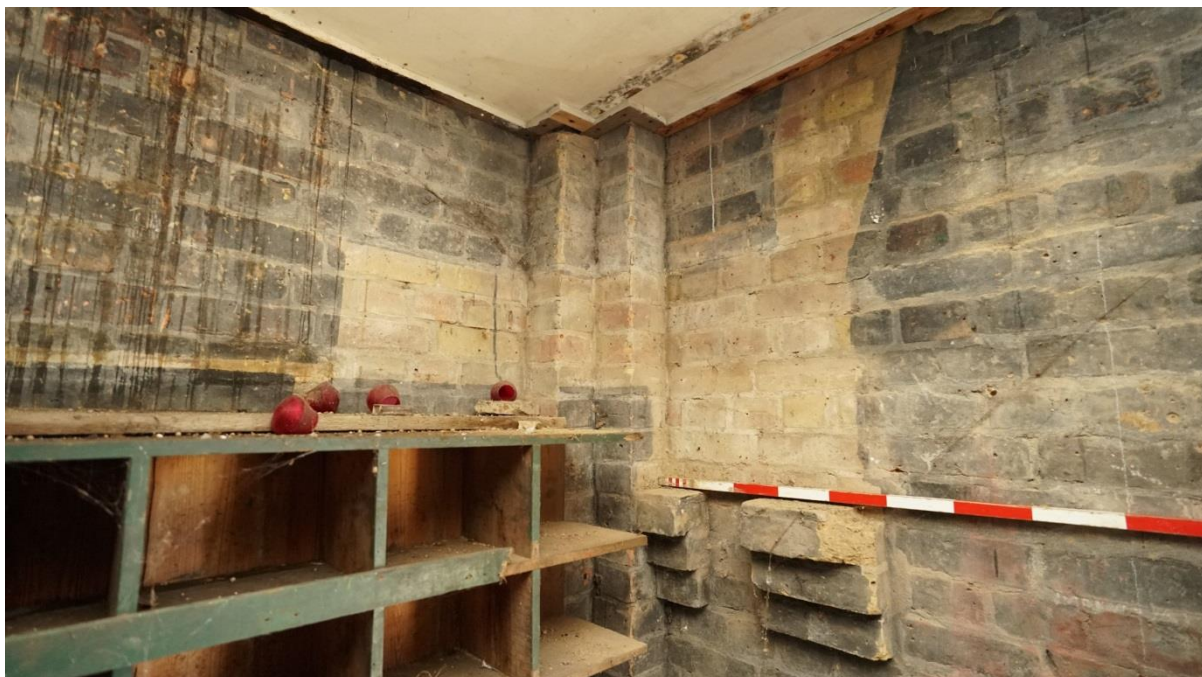
Plate 33. Interior of Building 2 – southern corner of the room with imprints of the half floor and ladder
